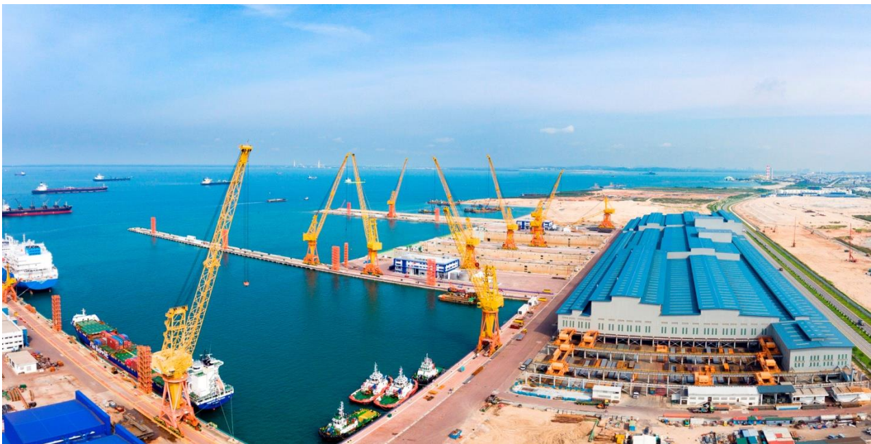
Southeast Asia's largest single solar rooftop at a shipyard will be installed atop Sembcorp Marine Tuas Boulevard Yard's steel structure fabrication workshop (building on the right with blue roof)
