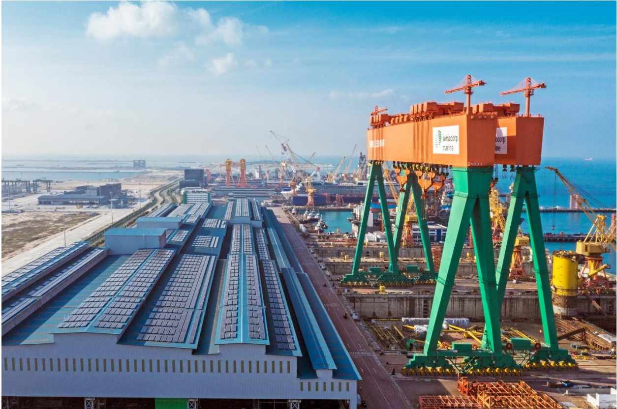
Solar panels (L) installed at Sembcorp Marine Tuas Boulevard Yard during Phase 1 of Sembcorp Marine and SP Power's collaboration
