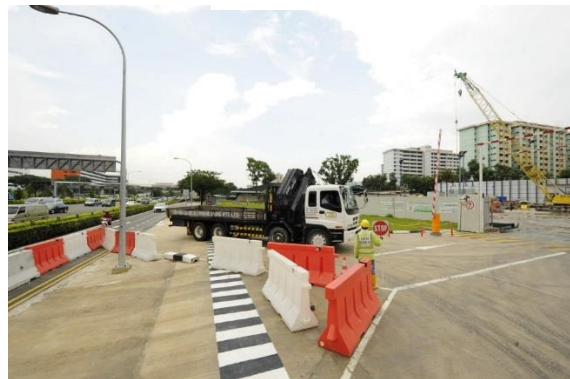
Heavy vehicle entering Kallang site through new access road
