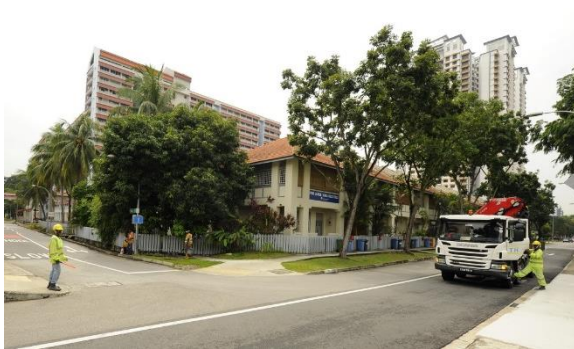
Vehicle commander boarding heavy vehicle to ensure it slows down approaching the site
