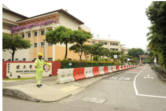
Water barricades to prevent jaywalking (May Road only)
