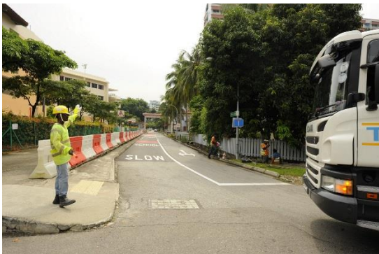
Marshal in place to direct traffic at the junction of May Road / Towner Road
