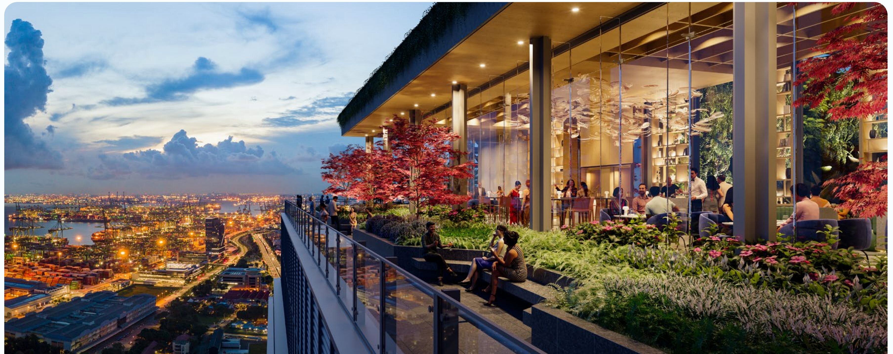
Labrador development: A landmark project featuring a Super Low Energy commercial tower and Southeast Asia's largest 230kV underground substation, exemplifying SP Group's commitment to grid reliability and sustainable energy solutions
