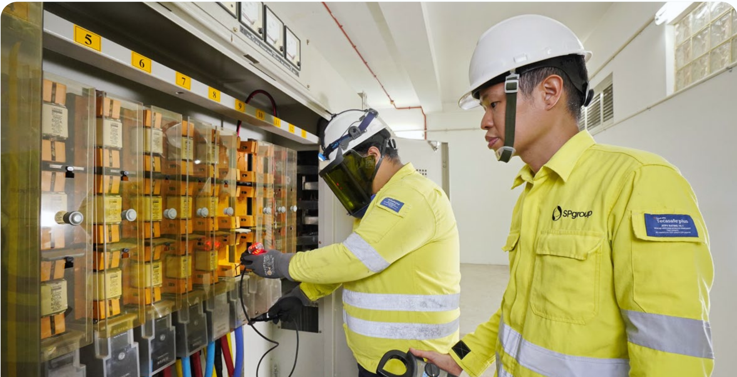
Safe work practices and proper use of personal protective equipment supporting safe operations
