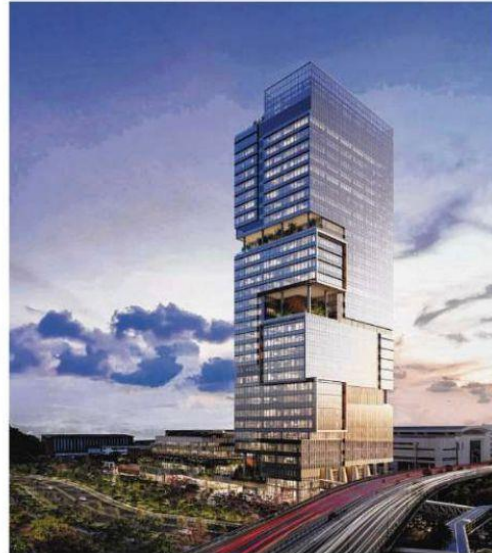
The thermal storage tank will be in the basement of the office tower of the Labrador Tower development. PHOTO: SP GROUP
