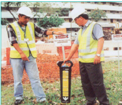
Fig. 3 - Cable detection Work and Cable Tunnels
