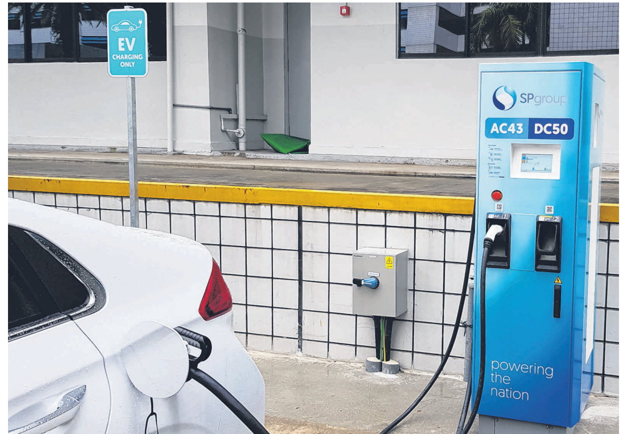
SP Group’s high-speed electric vehicle charging points, consisting of 19 43kilowatt (kw) alternate current chargers and 19 50kw direct current chargers, are able to charge a mid-sized electric car within an hour. ST PHOTO: CHRISTOPHER TAN
