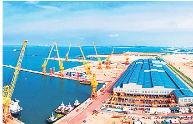
South-east Asia's largest single solar rooftop at a shipyard will be installed atop Sembcorp Marine Tuas Boulevard Yard's steel structure fabrication workshop (building on the right with the blue roof).
