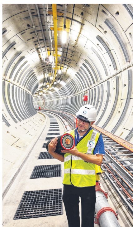
For most of their distance, the tunnels are 6m in diameter, about two storeys high, but at junctions, they swell to 11m, the height of about three storeys.
