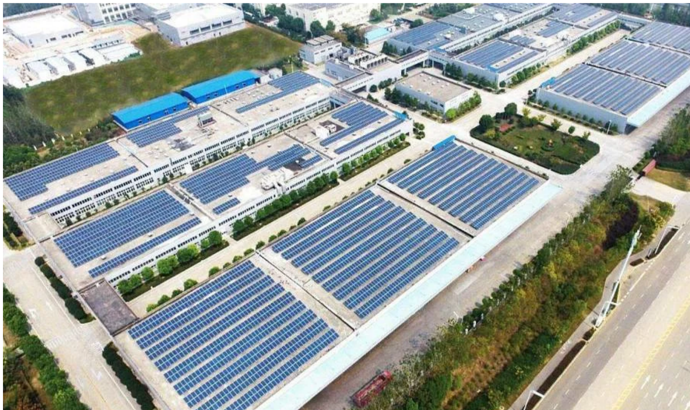
The rooftop solar panels at the Hefei Wahaha Group are one of the 50 industrial sites that were part of the first phase of the PV assets acquisition. PHOTO: SP GROUP
