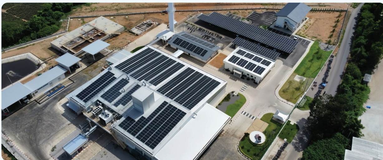
SP is expanding our solar PV footprint in Thailand, including Betagro's factory in northern Thailand's Lampang Province.
